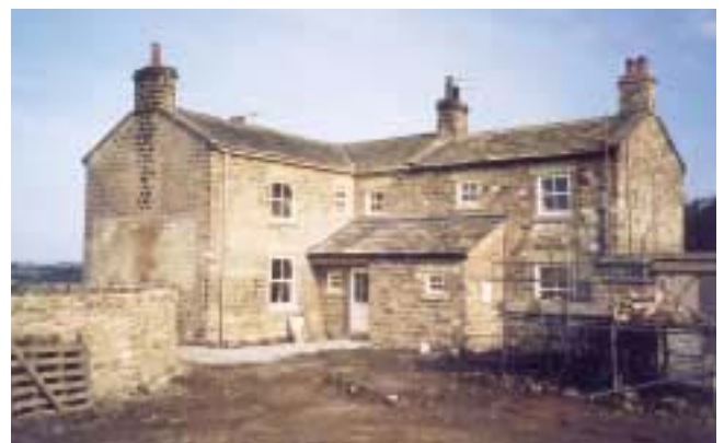
Field House during recent renovation
