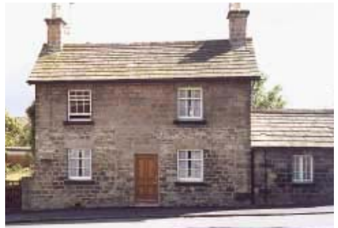
North View, Moor Lane
