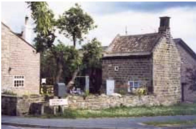
One-up, one-down cottage, Church Drive
