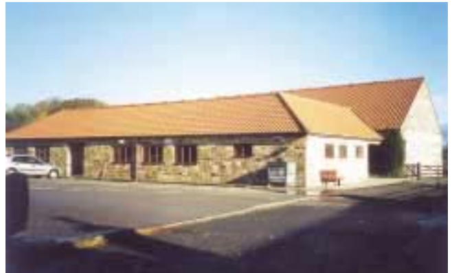
East Keswick Village Hall
