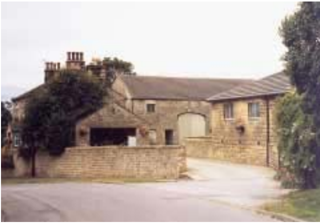
Manor House Farm, Moor Lane – c1800
